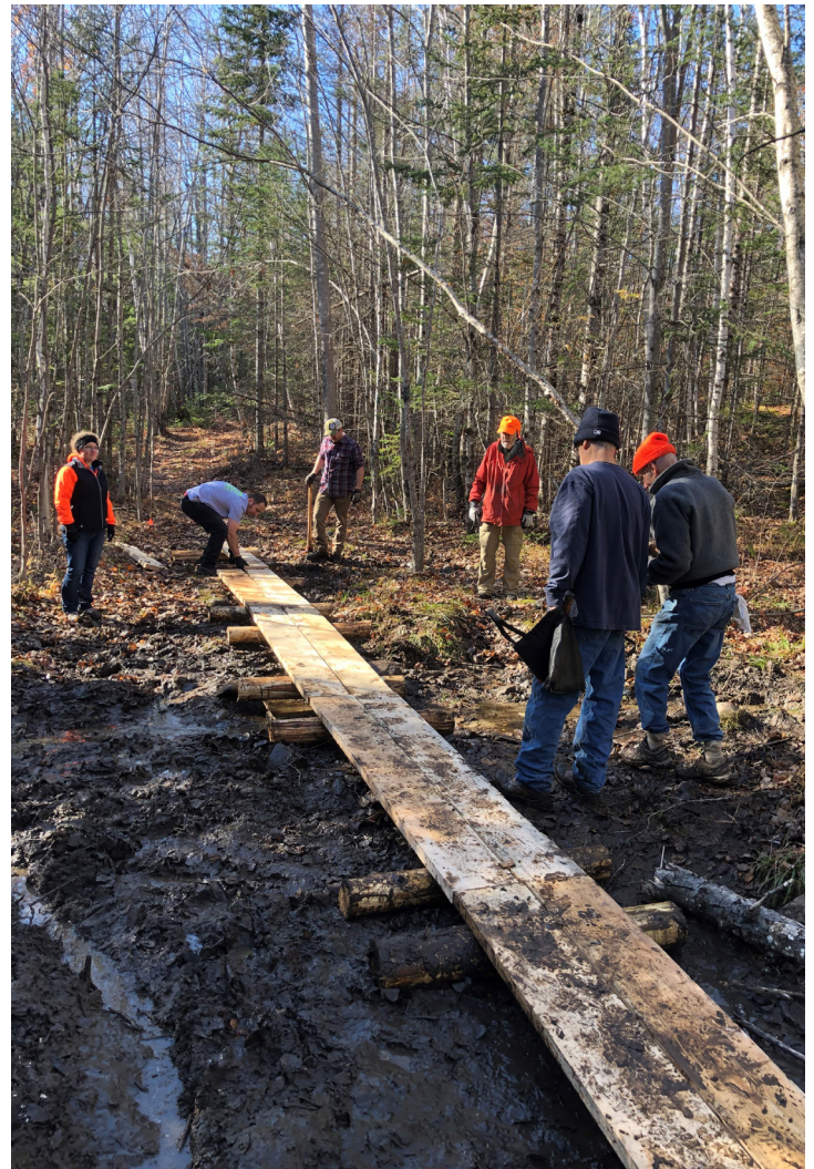
Bog boardwalk being built in Nov. 2021. photo by Geoff Gratwick.
